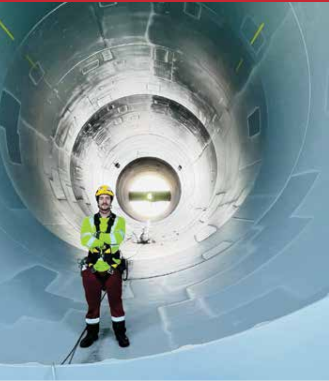
Local 56 member Brother Biel stands inside one of the Vineyard Wind turbine foundations.
